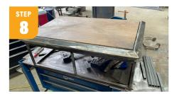
Tack weld the tubes to the frame of the tabletop. Be sure to keep the middle tube centered to allow the shelves to be symmetrical.
