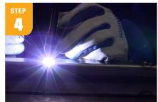
TIG weld the crush tubes in. Set Multimatic<sup>®</sup> 220 AC/DC for 100 amps and use .045" size ER70S-2 filler. Note that you need to cut the tubes to 176" instead of 2" so you have 1/6" weld step on each side. This will give extra weld strength when grinding the welds flush to the sides.
