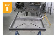
Using 1/8" 1x2 sq tubing for this part, cut 2 pieces 43" long with 45 degree cut on one end, a 28" piece with 45 degree cut on both ends, and one 26" piece. Be sure to debur your cut areas.
