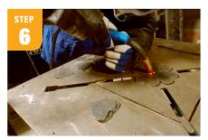
Weld four hearts together from the back side.
